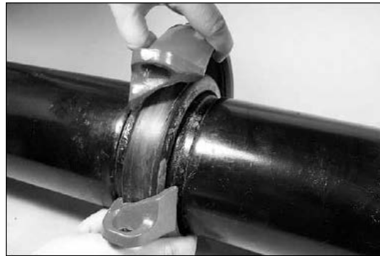
7. INSTALL HOUSINGS: Using the “swing-over” feature, install the housings over the gasket. Make sure the housings’ keys engage the grooves properly on both pipes/mating components.
