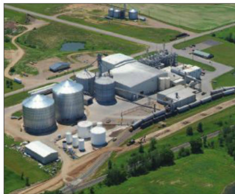
Photo courtesy of Ace Ethanol LLC Sweetwater will build its plant near the Ace Ethanol facility in Stanley, Wis.
