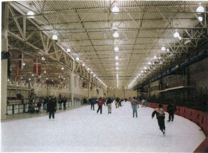
Plate 9. Metal halide lighting in industrial luminaires installed over this skating rink provides good general illumination for skaters and a glare-free ice surface. The uplight contribution creates a feeling of spaciousness and pleasantness in the space.
