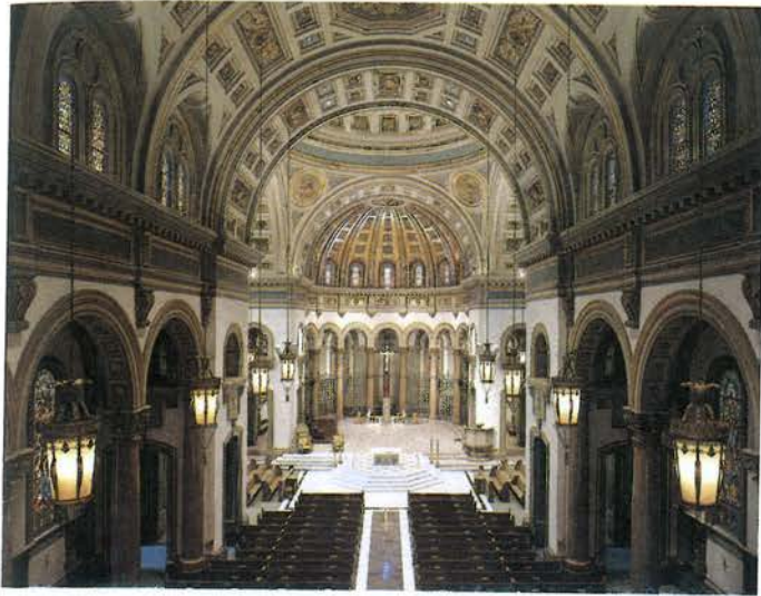
Plate 1. The magnificence of the architecture has been redefined by a new lighting system in this cathedral. Lanterns from 1929 were refurbished, 1949 downlights were retrofitted with tungsten-halogen lamps, a new indirect lighting system was installed to emphasize the ceiling vault and dome, and a television lighting system was added, all controlled to allow lighting level flexibility from 0 to 100%.
