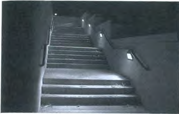
Figure 21-7. Effective hazard lighting on stairs. This lighting is unidirectional, emphasizing stair treads.
