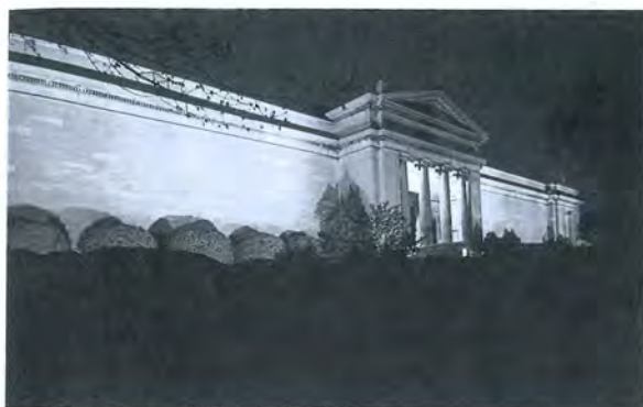
Figure 21-20. Good vertical surface illuminance without hot spots.
