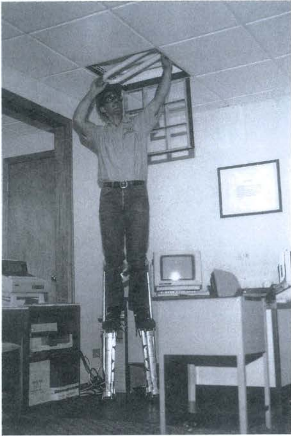
Figure 28-4. Stilts used for maintenance in spaces with low ceiling heights.
