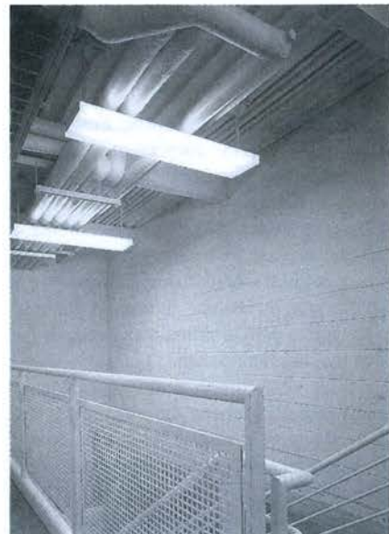
Figure 29-16. Adequate safety lighting must be used in spaces with obstructions or changes in direction or level, such as stairwells.
