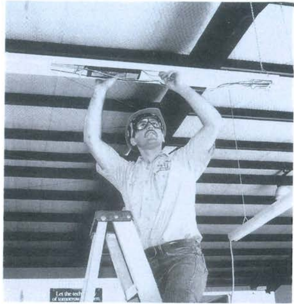
Figure 28-3. A ladder is used to change a ballast.
