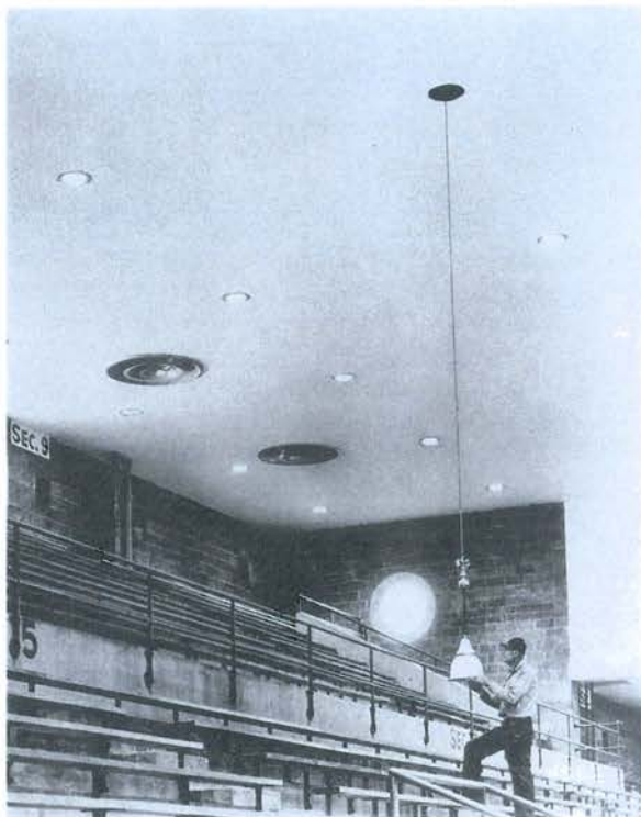
Figure 28-8. Disconnecting and lowering hangers.
