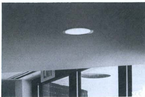
Figure 29-14. A ceiling soffit can block the line of sight to an exit sign.
