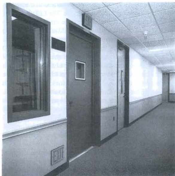
Figure 29-13. Supplemental exit signs mounted near the floor can be seen by occupants crawling along the floor in smoky conditions.
