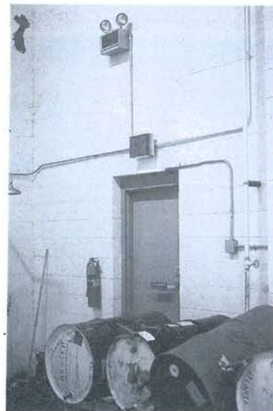
Figure 29-4. This wall-mounted sealed-beam unit provides emergency lighting for fire-fighting equipment (the fire extinguisher) as well as the exit approach that should be kept clear of obstructions (e.g., the barrels shown here).
