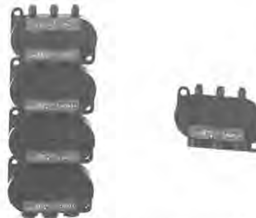
Figure 6.3 Averaging relay. (Courtesy of Johnson Controls Inc.)
