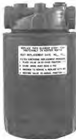
Figure 7.4 Charcoal filter. (Courtesy of Johnson Controls Inc.)
