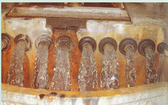
FIGURE S2: Nozzle outputs from the header tank in the Mahmud II Dam. (From Kâzım Çeçen, Sinan's Water Supply System in Istanbul , Istanbul Technical University/Istanbul Water and Sewage Administration, Istanbul, Turkey, 1992-1993, pp. 165-167. Reproduced with the permission of Istanbul Technical University, Istanbul, Turkey.)
