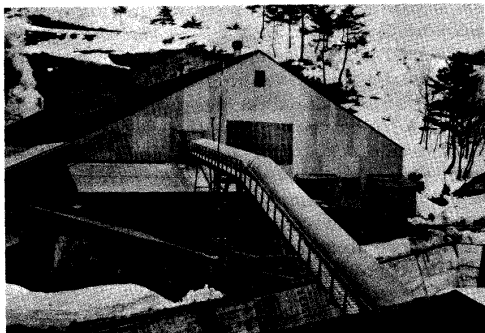
Figure 9.6 Zeolite plant at Itagaya, Japan. (Photograph courtesy of Professor H. Minato.)
