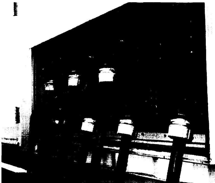
Figure 8—Bank of 19-tube connectors at the control house
