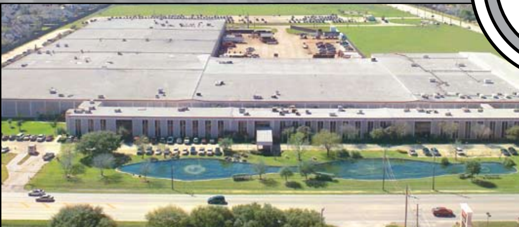
North American Headquarters & Manufacturing Facility (Houston, TX)
