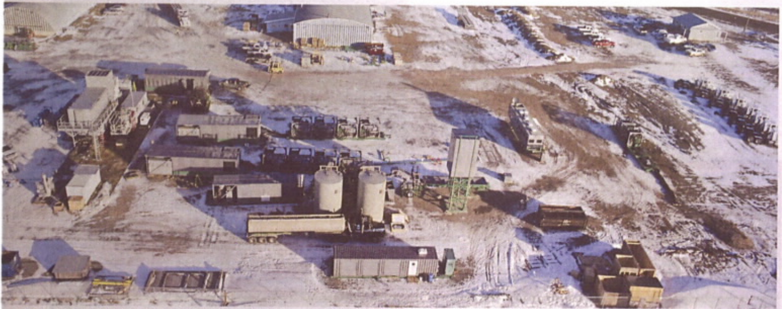
EVOLUTION WELL SERVICES HAS SET UP A DEMONSTRATION SITE IN LETHBRIDGE, ALTA., THAT BOASTS 20,000 HORSEPOWER OF PUMPING CAPACITY. A SIMILAR SITE USING CONVENTIONAL FRACKING ASSETS WOULD BE DOMINATED BY 10 TRACTOR TRAILER PUMPS.
