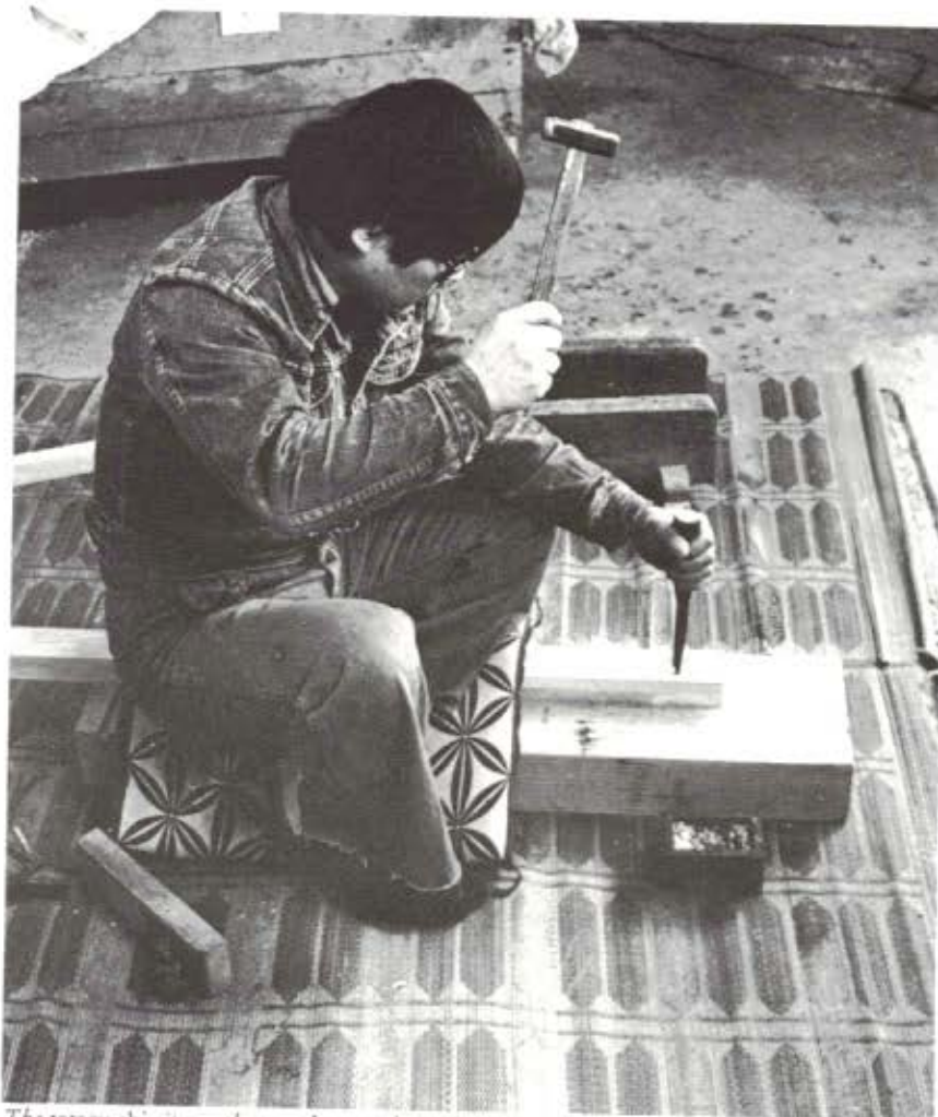
Fig. 9: Mortise chisel/chopping method
