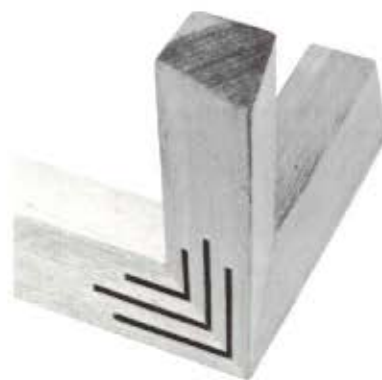
Three variations of the decorative splined mitered joint. Piece with angled faces, at right, is the most difficult of the three to make.
