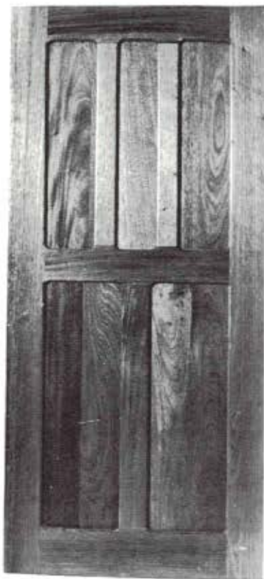
Routed sticking stops short of corners in raised-panel door, left, but continues around corners of flat-panel door, center. Both are Honduras mahogany. Detail from oak door, above, shows routed sticking combined with molding.
