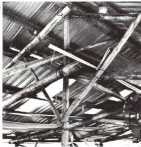
Brackett's pole-and-wire shop is spacious and well ventilated; detail, left, shows cross-bracing at central post.
