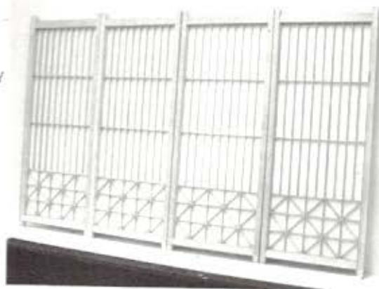
The lattice structure of the shoji can be organized in various ways and is covered with rice paper. Above are common (ma) shoji; at right, tokonoma shoji.
