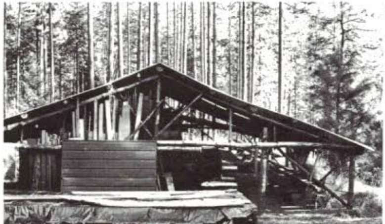
Brackett's pole-and-wire shop is spacious and well ventilated; detail, left, shows cross-bracing at central post.
