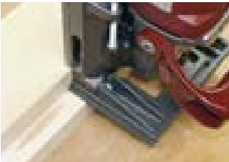
Repair in the groove
