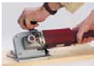
Planing protruding patch
