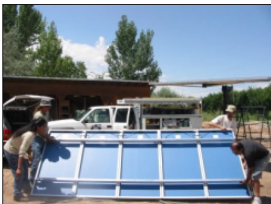
Sub-Array Approach. Requires a lot of people power. Lift by the tracker rails only, not the module frames!
