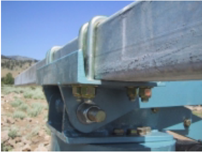
TIGHTEN NYLOCK 5/16" U-BOLT NUTS EVENLY .
