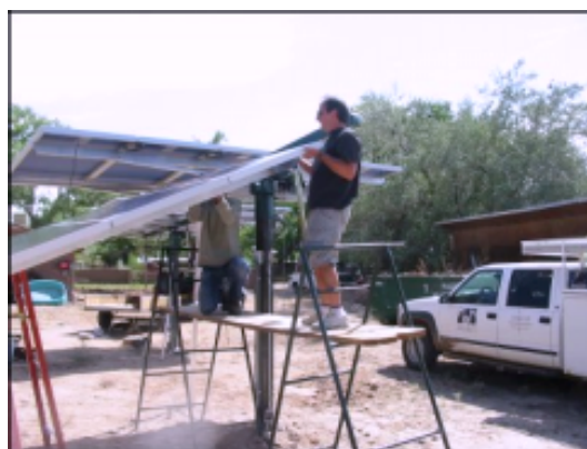
Lifting and bolting the sub-array onto the tube. Typically a 3-person job: 2 lifters, 1 bolter.
