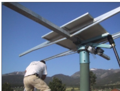
One installer, one piece at a time approach. Modules are being used to "square-up: the frame.
