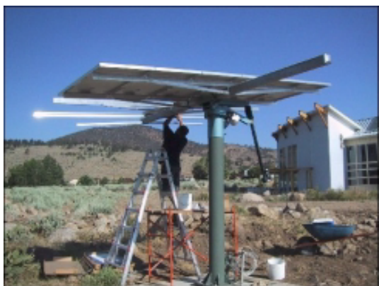
Sub-Array Approach. Requires a lot of people power. Lift by the tracker rails only, not the module frames!
