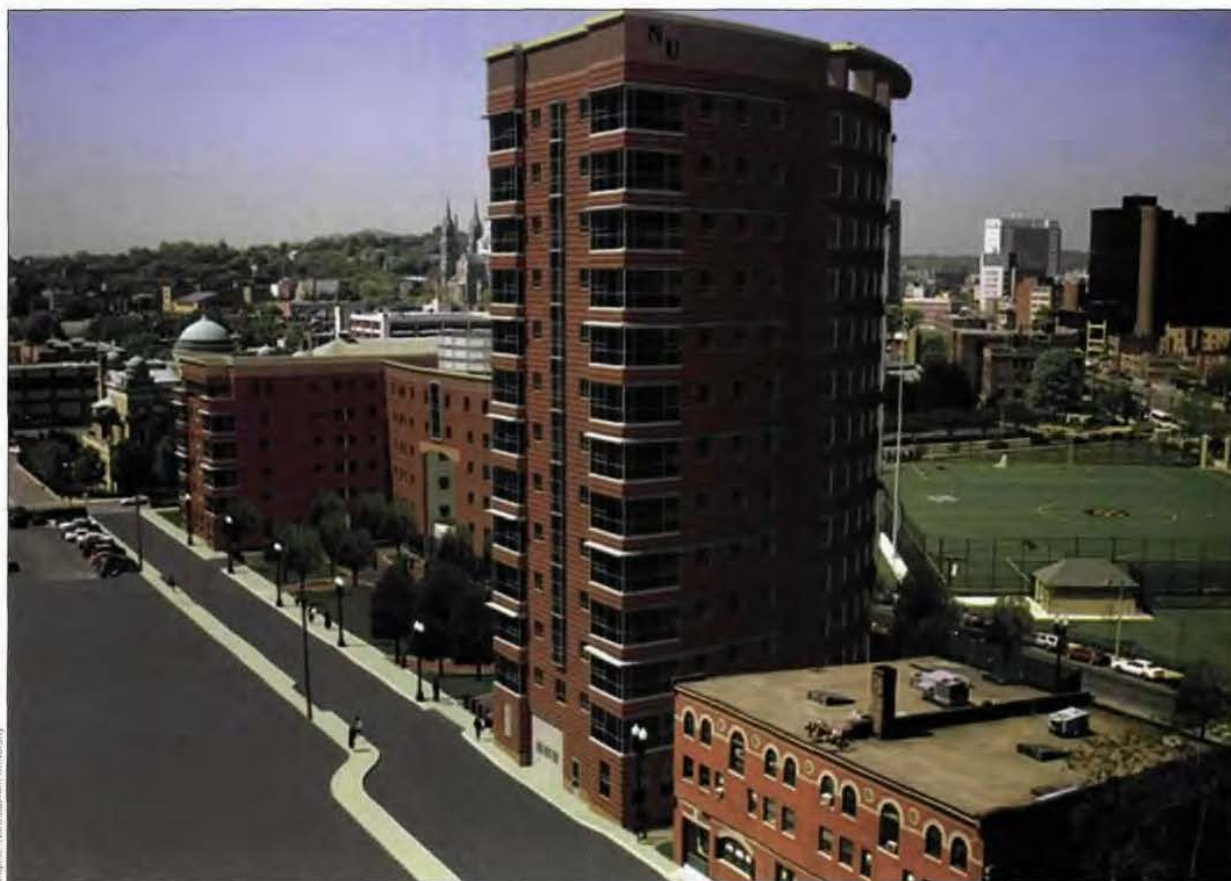
The new dorm, which will house 600 students, will be fully sprinklered and will contain smoke alarms in both the public areas and the individual units.
