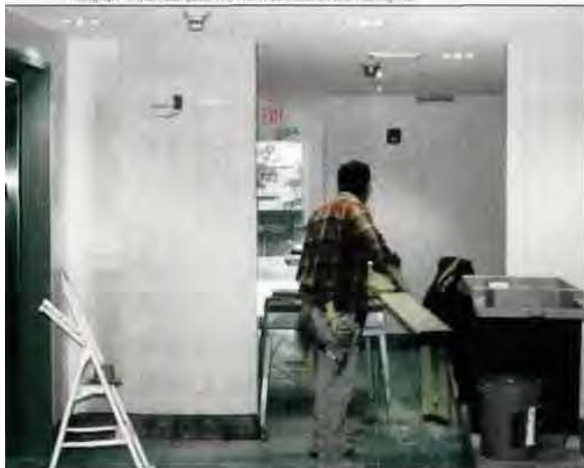
Early installation of smoke detectors is the primary cause of nuisance alarms.
