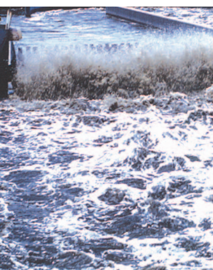
Brush Aerators in an Oxidation Ditch
