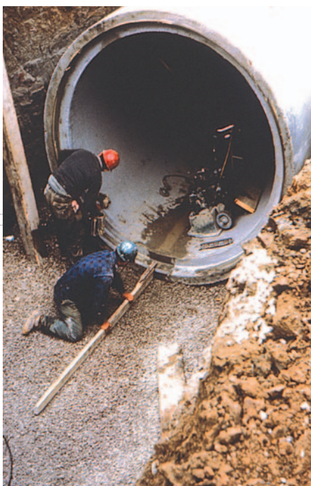
Workers install sewer line
