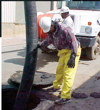
Sewer line maintenance
