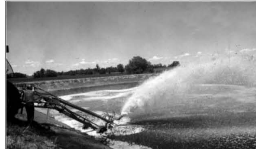
Figure 11. This PTO-powered, high-capacity pump can either fill tankers or bypass effluent to agitate a lagoon, or both.
