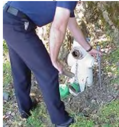
Ground sloughoff prevents full turning of the spanner
