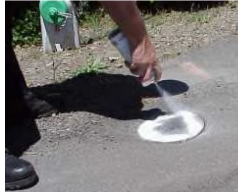
Painting a gate pot which had been covered with "slurry seal"
