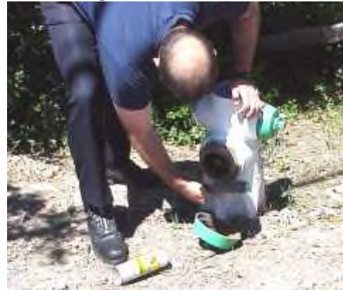
Cleaning threads with a wire brush
