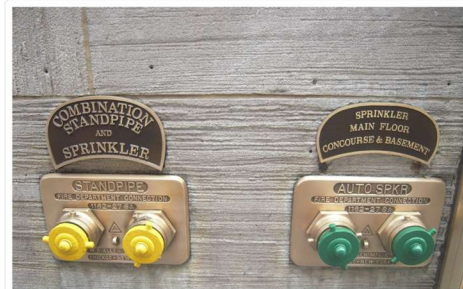
Fire House, Warehouse complex, Active fire protection (AFP) standpipes
