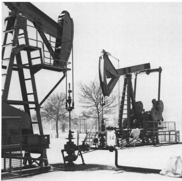
Figure 3.66 Surface pumping units in the Schoonebeek oil field, the Netherlands. (Photo: NAM).
