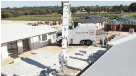
Robot Bricklayer Can Lay 300 Bricks an Hour
