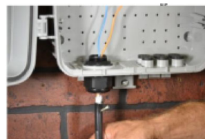
Figure 10 Routing Feed Cable Through Port Plate
