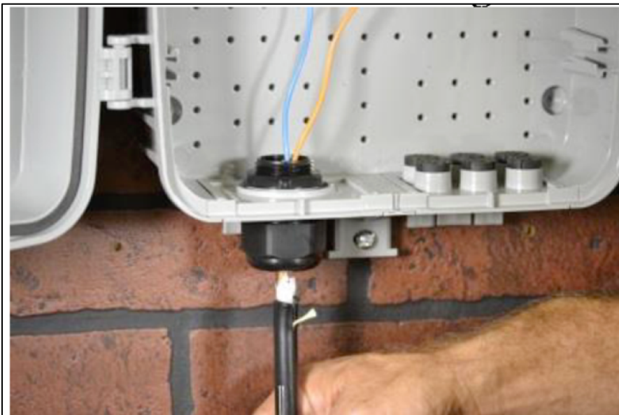
Figure 10 Routing Feed Cable Through Port Plate
