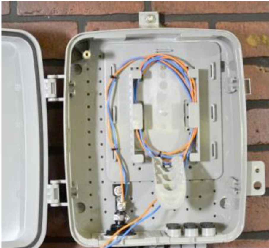
Figure 16 Complete Buffer Tube Routing
