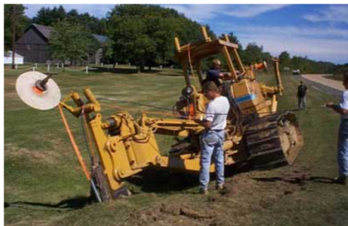
Plowing in direct buried cables (L) and directional boring (R)
