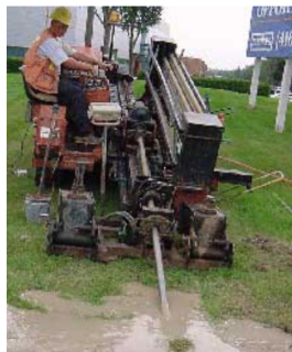
Plowing in direct buried cables (L) and directional boring (R)
