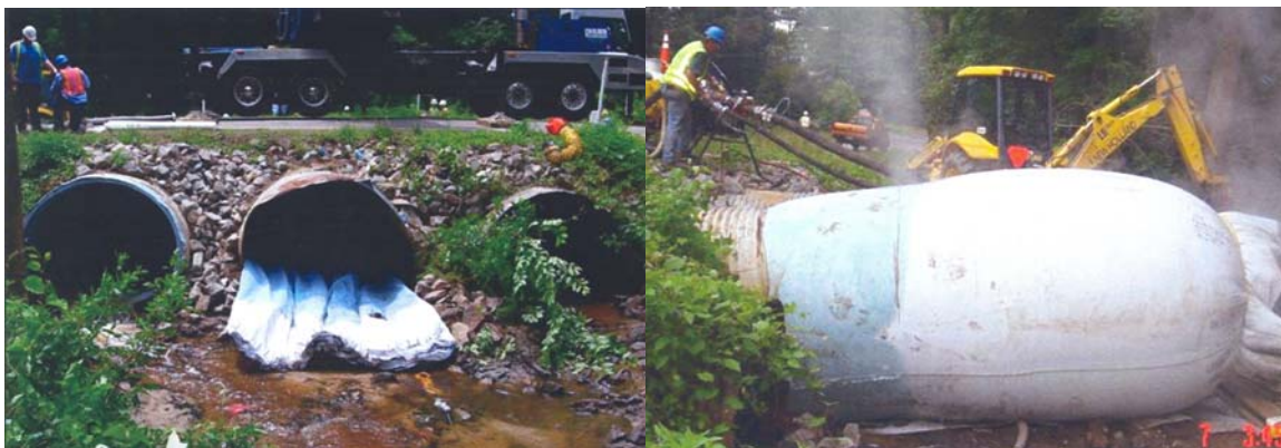
Figure 3-3 Pull and Inflate process (NASSCO, 2007).
