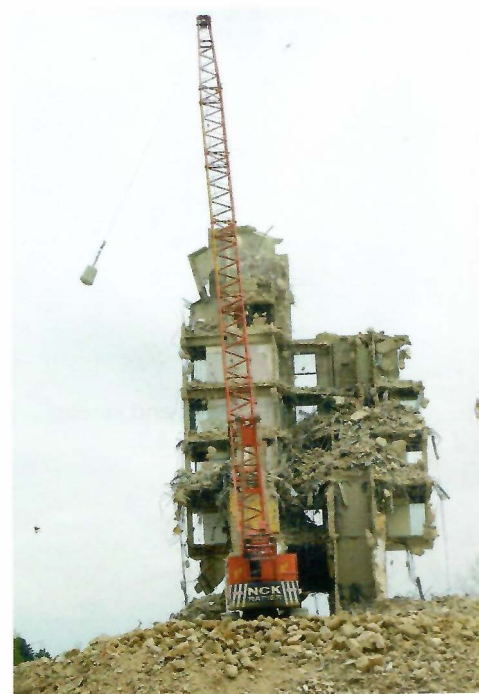
▲ FIGURE 5.10 Kinetic energy and work A moving object, such as a wrecking ball, processes kinetic energy and can do work. A massive ball is used in demolishing buildings.
