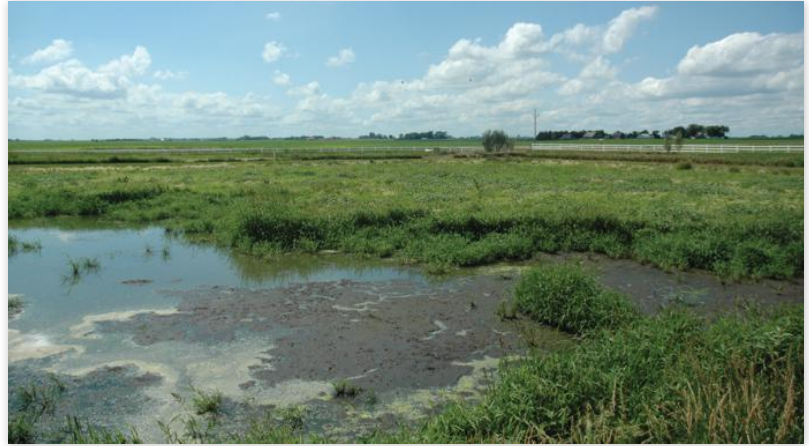
The liquid from the settling basin is released to a VIB (vegetative infiltration basin), which is a series of tiles with grasses growing on top. Contributed photo
