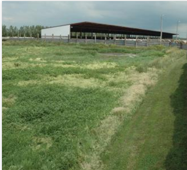
As the liquid passes through the VIB, it's filtered naturally through grasses (brome and canary grasses) and approximately 50 percent of the nutrients are absorbed. Contributed photo
