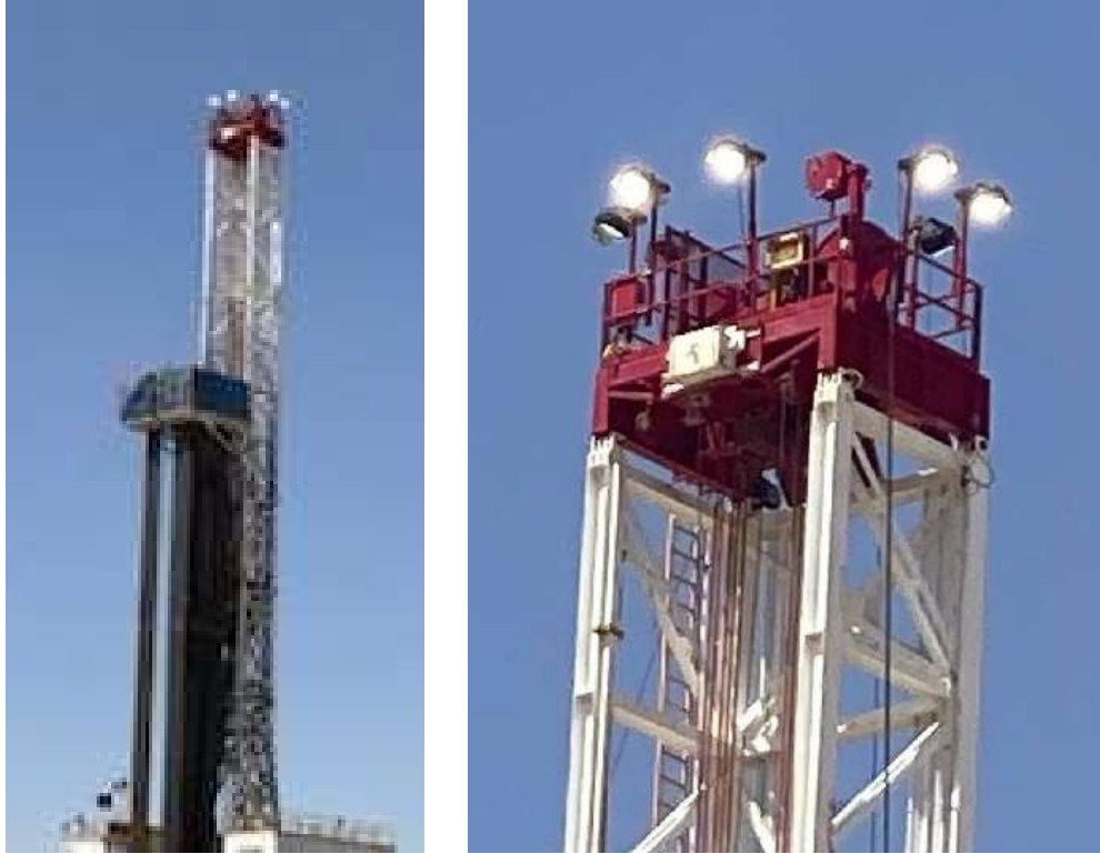
Fig. 1: Ensign 774 with non-C&M lighting system (photo taken on or about Mar. 15, 2022).
