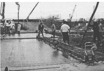
Figure.3 Removable rails, double width strip
