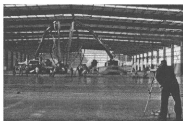
Figure.6 Two concrete pumps, optical levels
