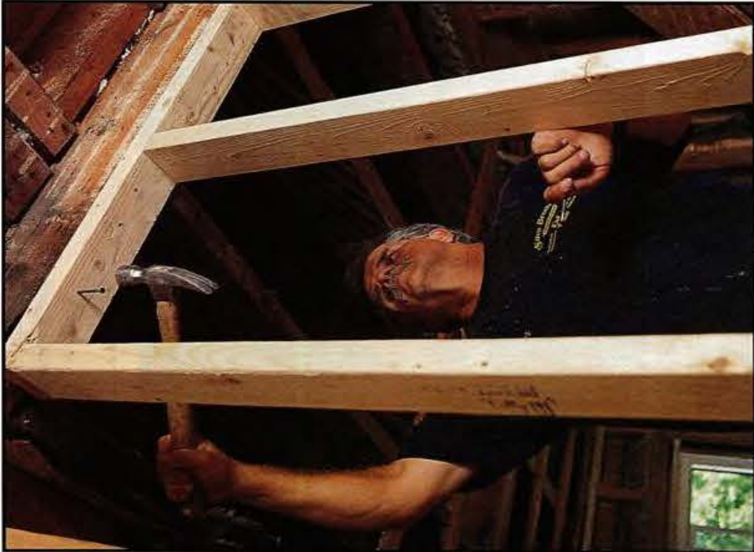
Although building codes allow walls that don't bear loads to be framed with studs spaced 24 inches on center, Tom Silva installs his studs 16 inches on center because that makes for a stiffer, stronger wall.
