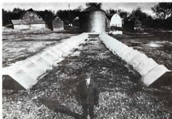
Kern'l Komfort solar collector produces upwards of 300,000 btu's of free heat per hour, which is equivalent to saving about 4 gals. of LP gas per hour.
