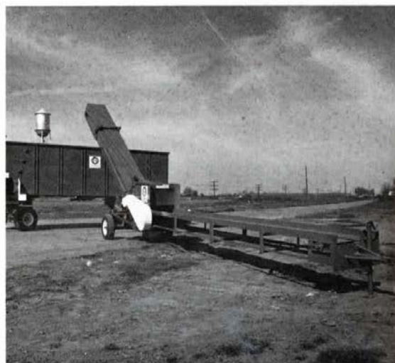
A water applicator is standard on the Crose portable baled hay slicer. Molasses applicator and pump are optional.
