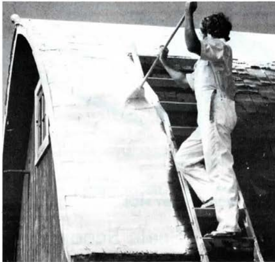
Rapid Roof was applied directly over the existing, badly-worn asphalt shingles on this barn roof.
