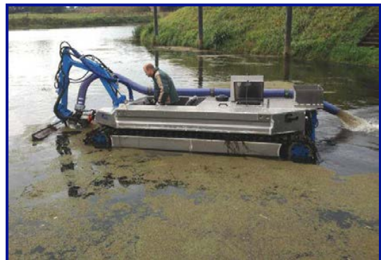
Suction an pumping of swimming algae and weeds
