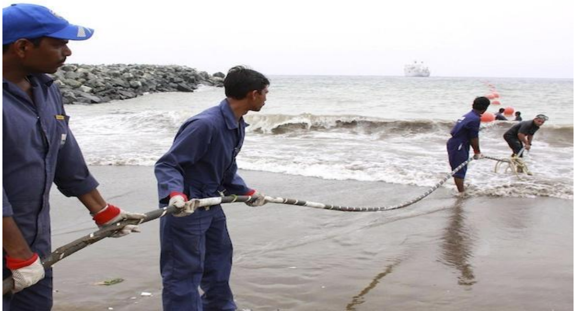
Figure 5.4.: Laying of Submarine cable
