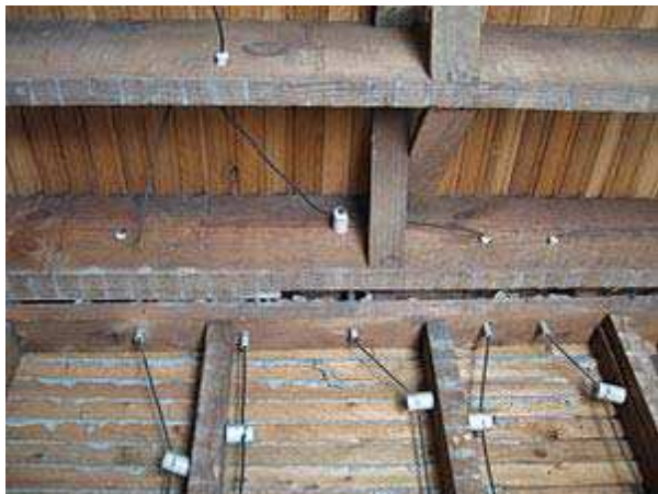
Fig. 12. Knob and tube wiring in a 1930 home. View looking upwards at upper wall stud bays and nearby ceiling joists [24].
