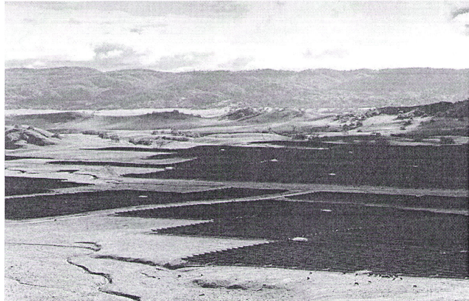
Capital Dynamics and First Solar completed the 280-MW ac California Flats Solar Project. Hearst
