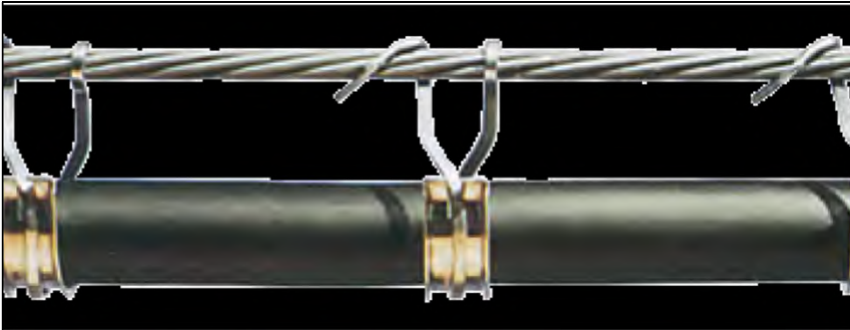
Figure 5: CAB Cable Rings and Saddles Installation
