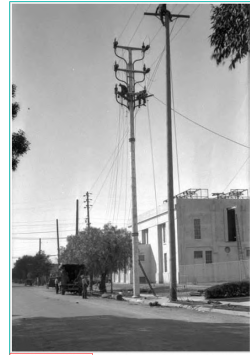
(1930s)* - View of the first steel pole installed on Bureau of Power and Light system, it appears to be standing in front of a distribution station.
