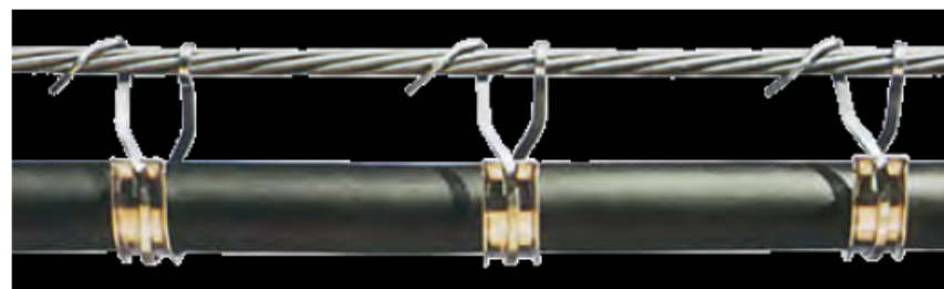
Figure 5: CAB Cable Rings and Saddles Installation
