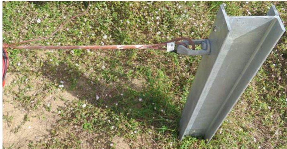
End-pier Kit (and example installation)
