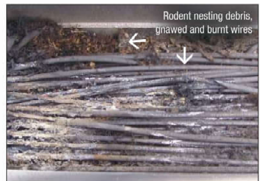
Rodent nesting in tray causes fire and system shutdown.
