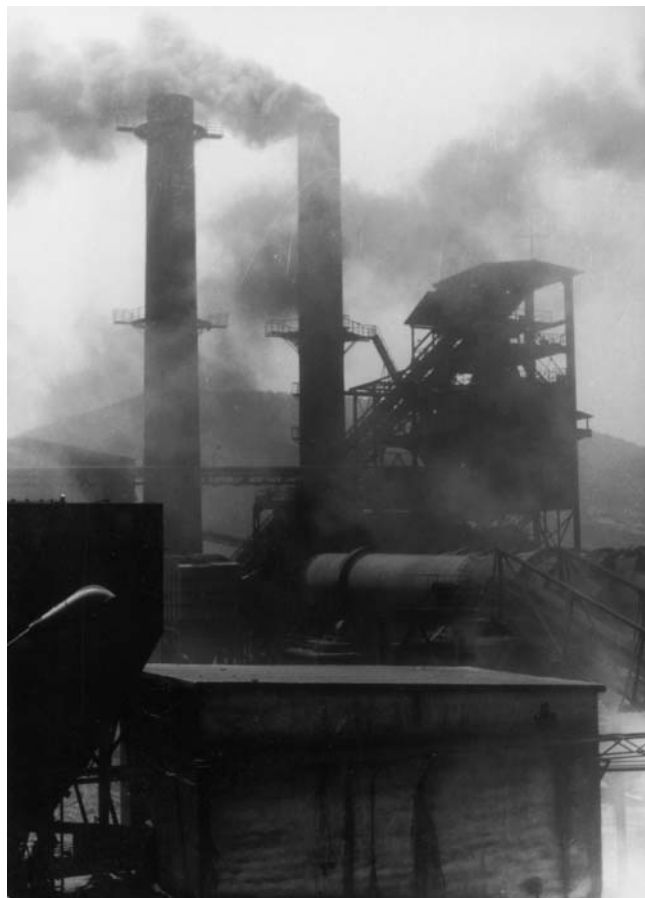
Fig. 8.1 Example of an industrial plant (pyroprocessing of minerals) heavily polluted with airborne particulate solids
