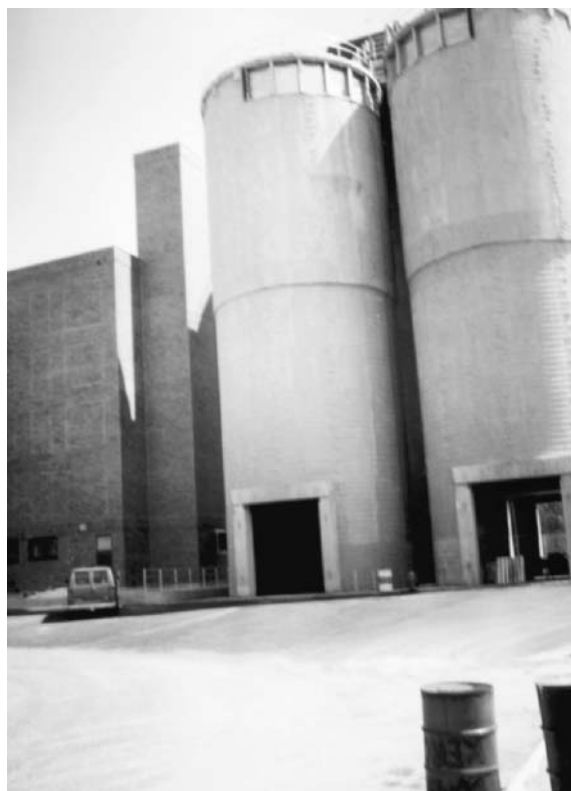
Fig. 8.45 Photograph of the outside product storage silos at OCUA (courtesy Ocean County Utility Authority, Toms River, NJ, USA)
