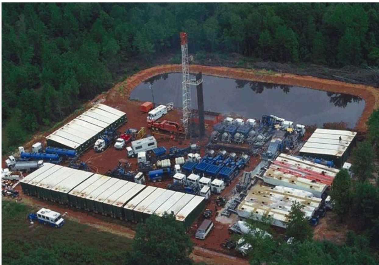
Figure 12 Large scale treatment, carried out on several low permeability zones simultaneously.
