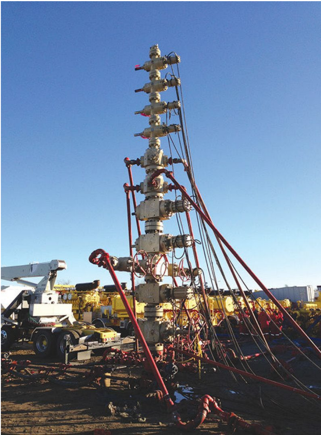
Figure 15 A “frac stack” atop BP’s D-1 well in Oklahoma’s Woodford shale while the well was being refractured in early 2013. BP doubled production from horizontal shale gas wells last year in a program meant to determine if refracturing
