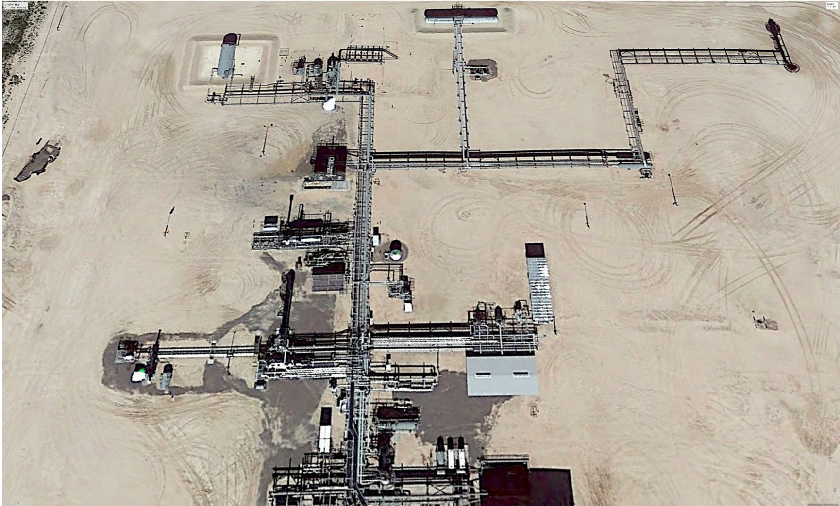
EX2075, Google Earth Image – Chevron Mabee CO2 Recycle Facility (10/4/2014) (after addition of NGL Recovery Plant).
