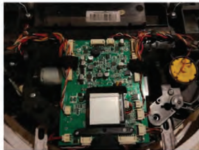
Motor Control DCDC BMS
