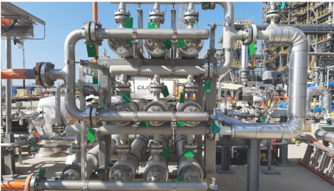
HISELECT® powered by Evonik membrane unit for hydrogen in Texas, United States of America
