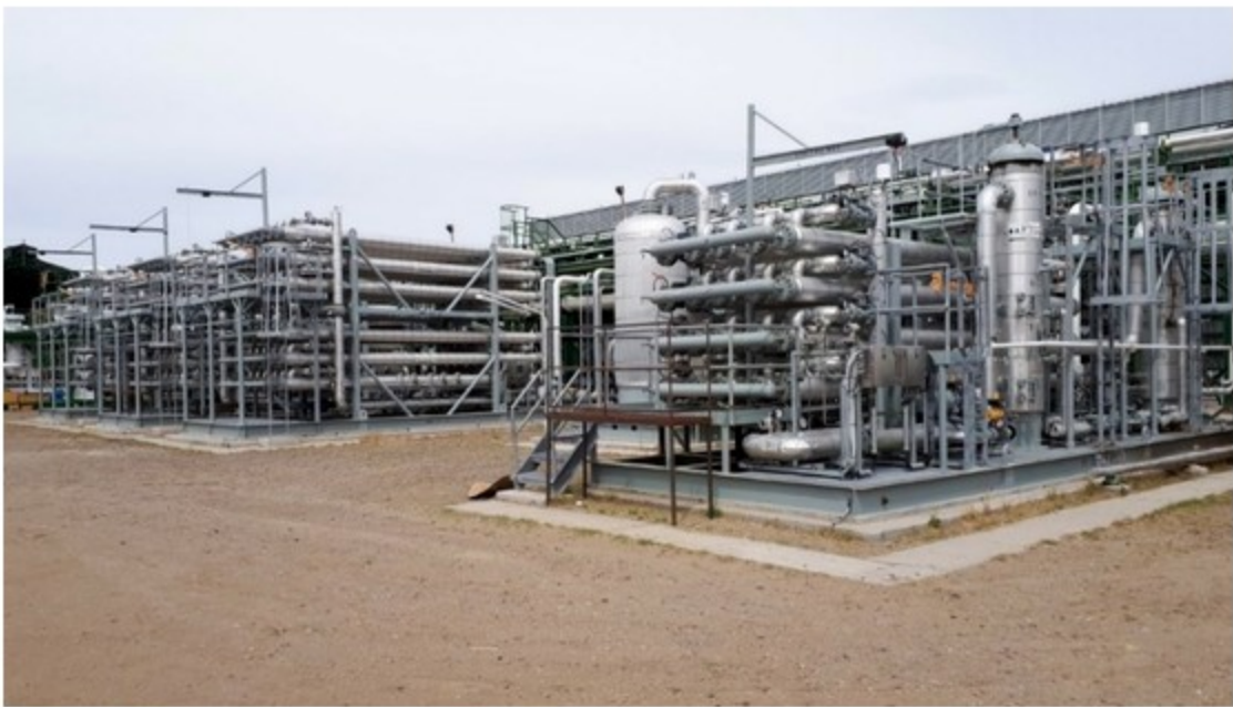
HISELECT® powered by Evonik membrane cartridges for natural gas, South America
