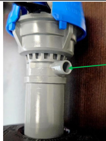
bowl fill valve outlet port
