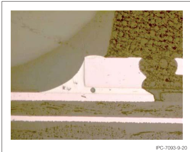
Figure 9–20 Side fillet on bottom termination component good wetting to copper lead.
