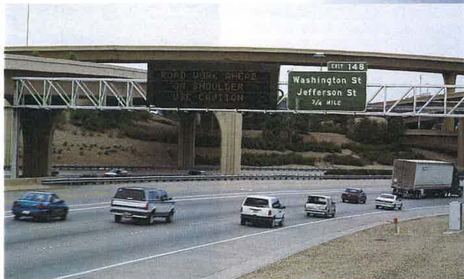
Advanced traffic and freeway management systems use monitoring, information-gathering, and control (automation) strategies to improve traffic flow. This variable message sign, for example, provides real-time information to drivers about incidents, alternative routes, and safety.
