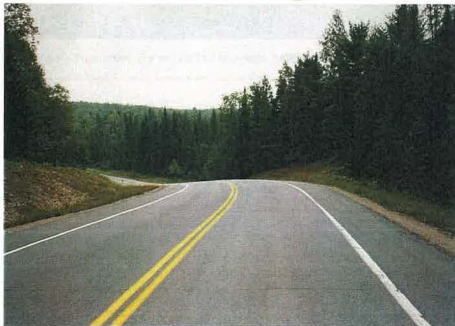
A typical two-lane rural highway.
