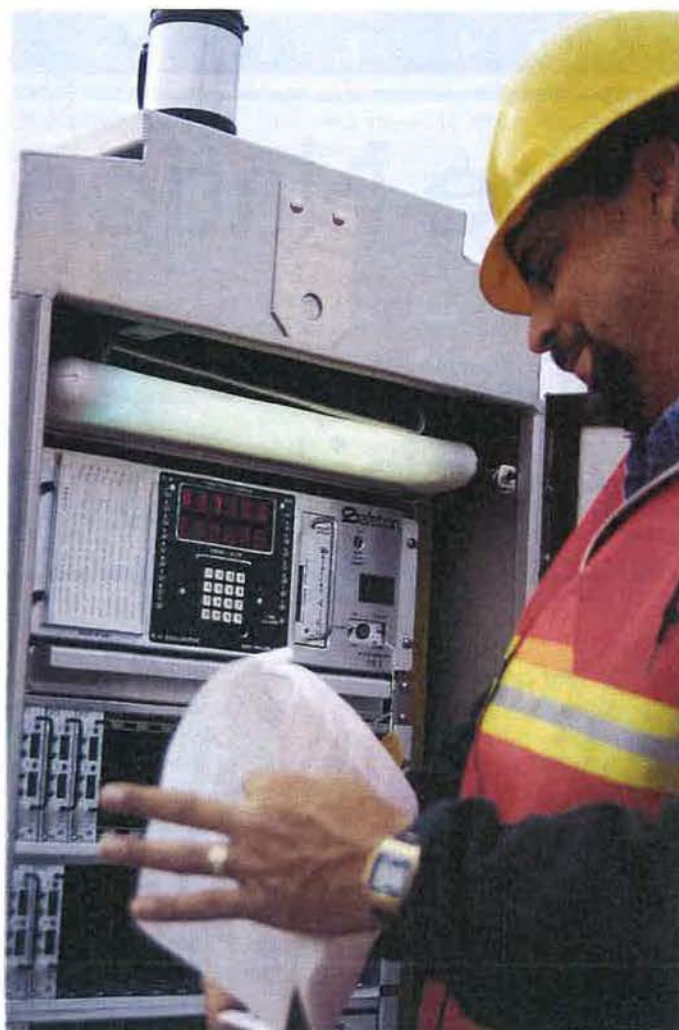
A worker tests the communications equipment that transmits traffic volume, average speeds, and video images of the traffic on Interstate 10 to the traffic operations center in Phoenix. Communications networks are among the fundamental structural elements that make up ITS infrastructure.
