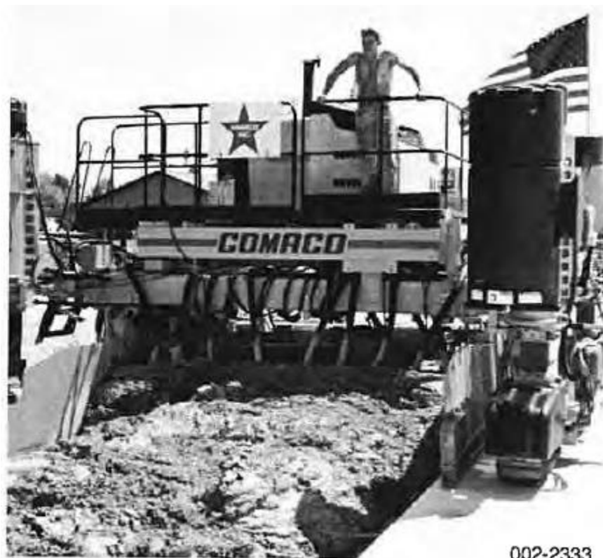
Concrete spread evenly in front of machine
