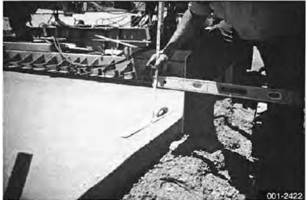
Check concrete grade
