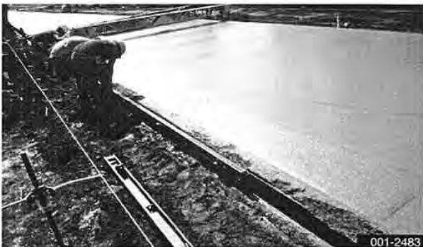
Placing forms behind a driveway curb
