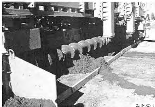
Paving over final header
