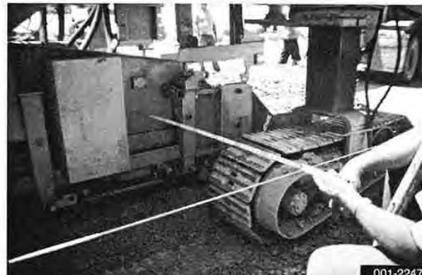
Measure offset between line and form
