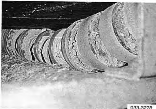
Concrete build up
