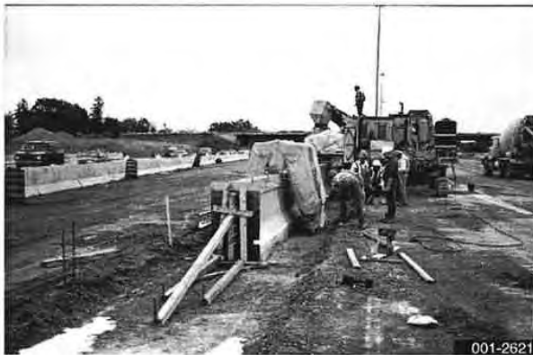
Vibrate concrete around header
