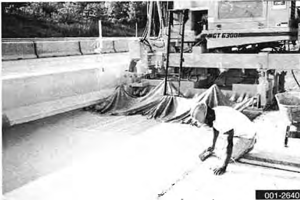
View of minimum clearance paving
