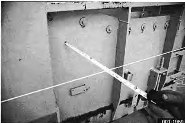
Measure offset distance (left guideline)
