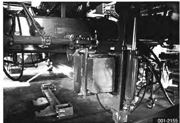
Install conveyor support beam
