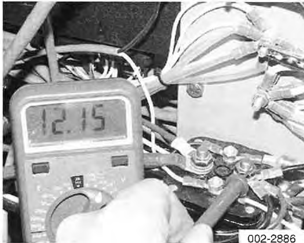
Check power relay voltage
