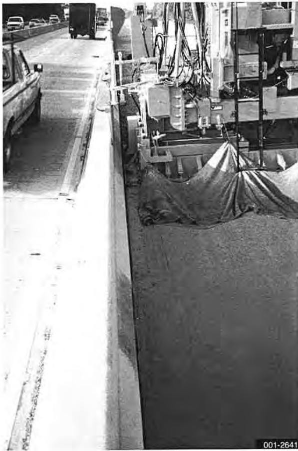
View of minimum clearance paving
