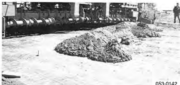
Machine set behind header
