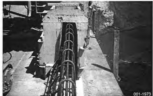
Check cage steel entering form
