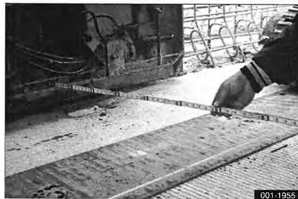
Measure offset distance (guideline under machine)
