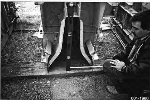
Adjust slope of barrier wall
