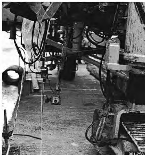
Adjust sensors to guideline
