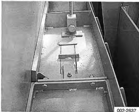
Remove cover plate in top of form
