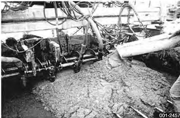
Placing concrete in front of the mold
