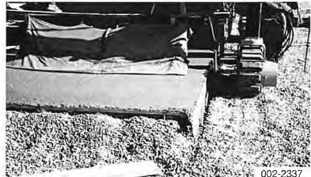
Finish concrete around header
