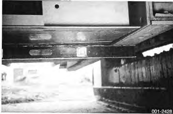
Straightedge From Main Pan Under Sideplate
