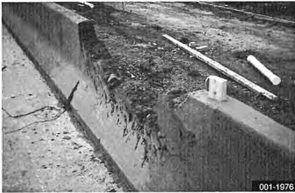
Concrete set up in form
