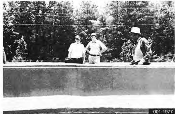
Example of concrete slump variance
