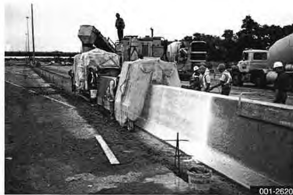
Spray the wall with curing compound
