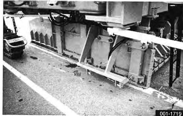
Machine in Position on Edge of Slab
