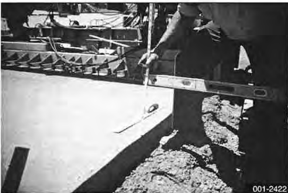
Check concrete grade
