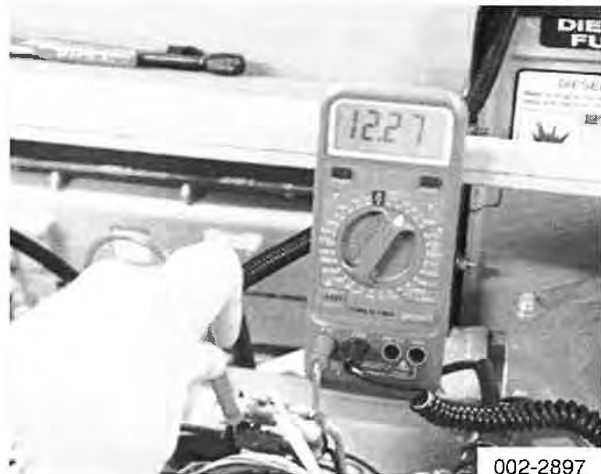
Check low oil pressure relay
