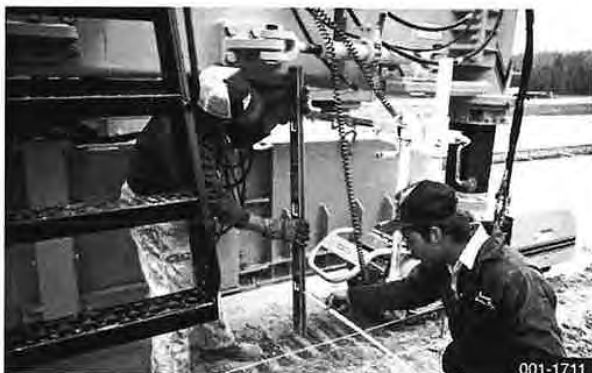
Measure offset between line and frame
