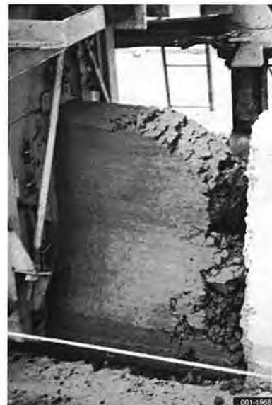
Back form against existing wall
