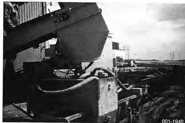
Swing conveyor into position
