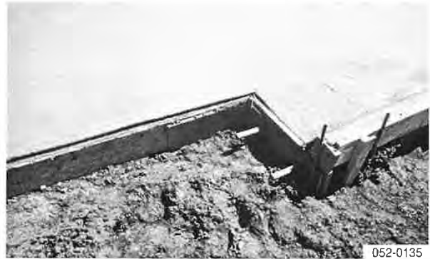
Box out for intersection tie-in
