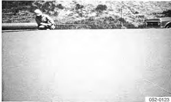
Check crown with stringline
