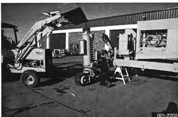
Remove rear leg for minimum clearance paving
