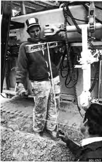
Measure grade between line and frame
