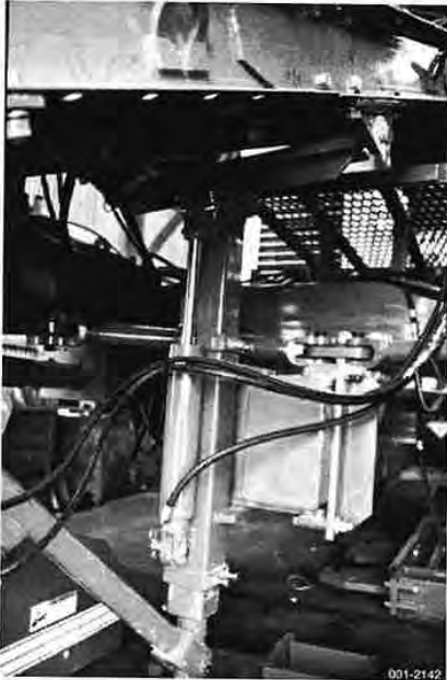
Install conveyor supports
