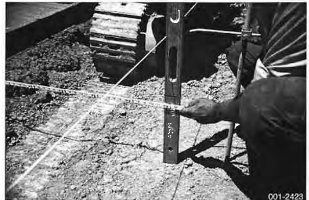
Check concrete offset
