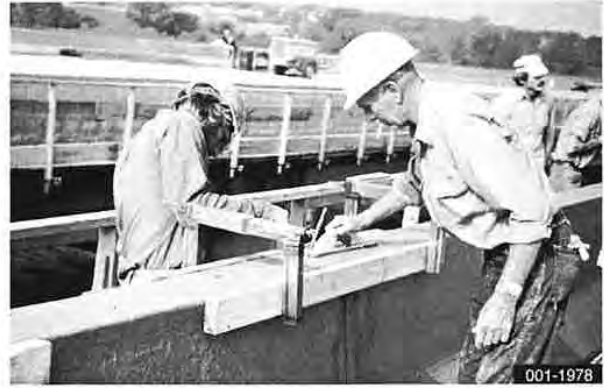
Setting repair forms
