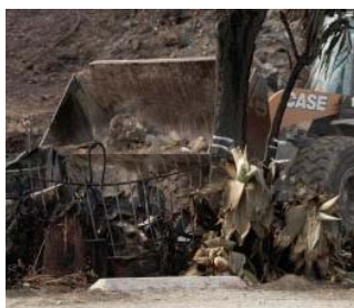
Caltrans Starts Repairs to Road Infrastructure Ravaged By Wildfires
